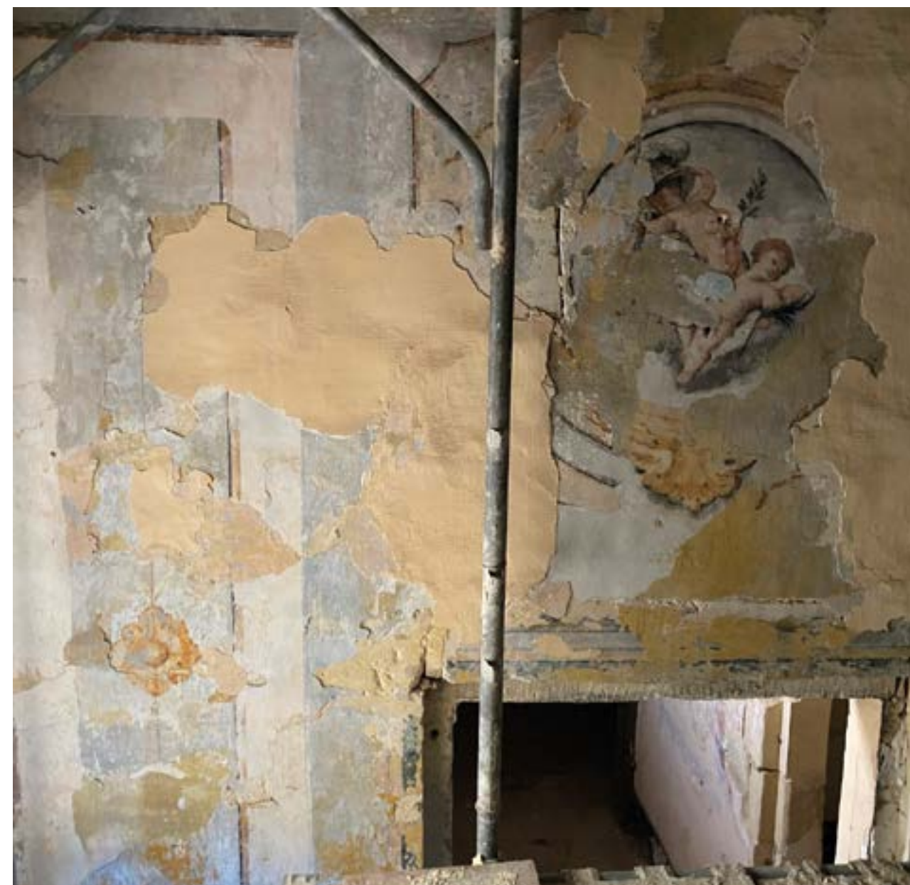
Detail of the internal wall paintings at the NBC Palazzo in Old Mint Street
