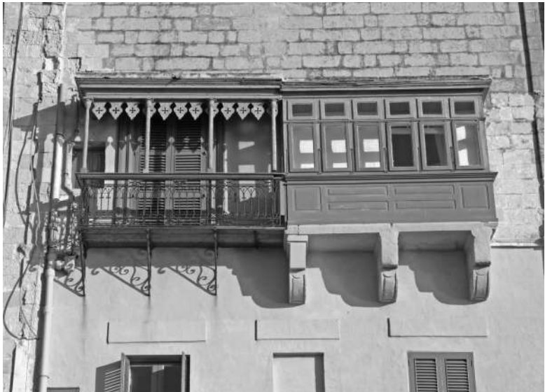
A closed balcony with an adjacent timber-floored counterpart.
